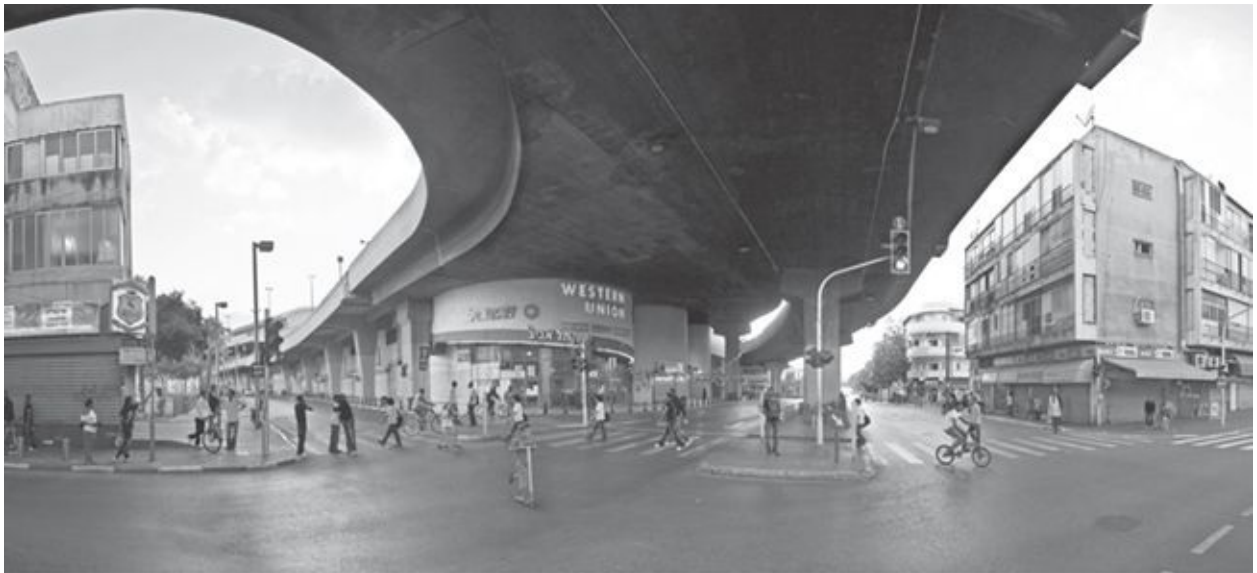
Bus platforms making their way through Neve Sha'anun to the New Central Bus Station: view from Levinsky Street. Photograph: Roi Boshi.
