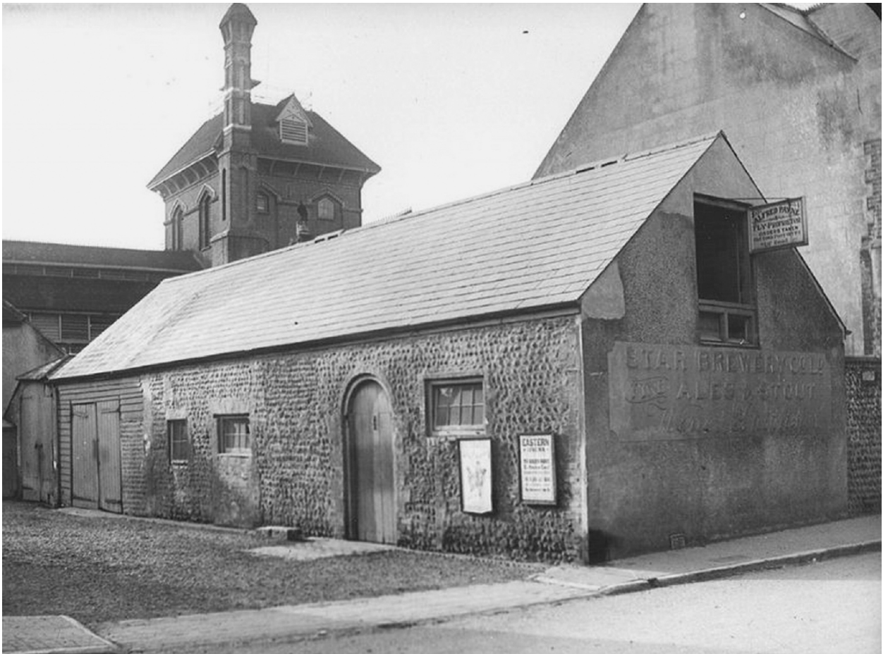
39. Star Brewery, Eastbourne, Sussex. This was the HQ of what is believed to be a Section VII sabotage and intelligence cell, operating throughout the war from March 1940. A wireless set was hidden in the brewery chimney. (East Sussex County Council Library & Information Service)
