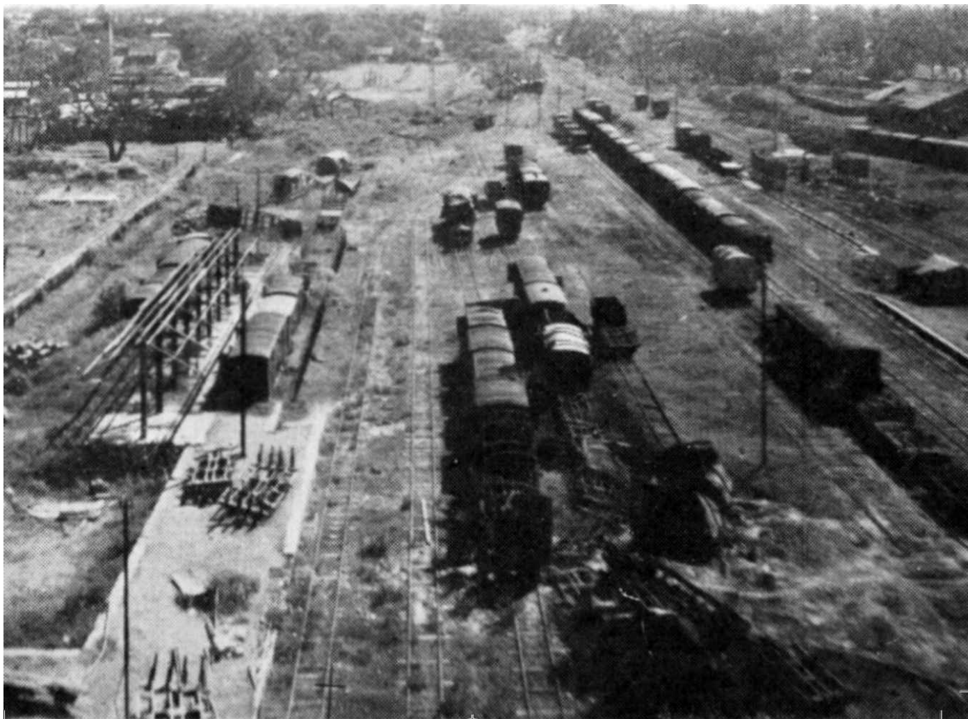
A low-level oblique photograph showing the extent of the damage caused by Allied air attacks on the town and railway junction of Pyinmana in central Burma. Much wreckage of rolling stock can be seen throughout the sidings. (HMP)
