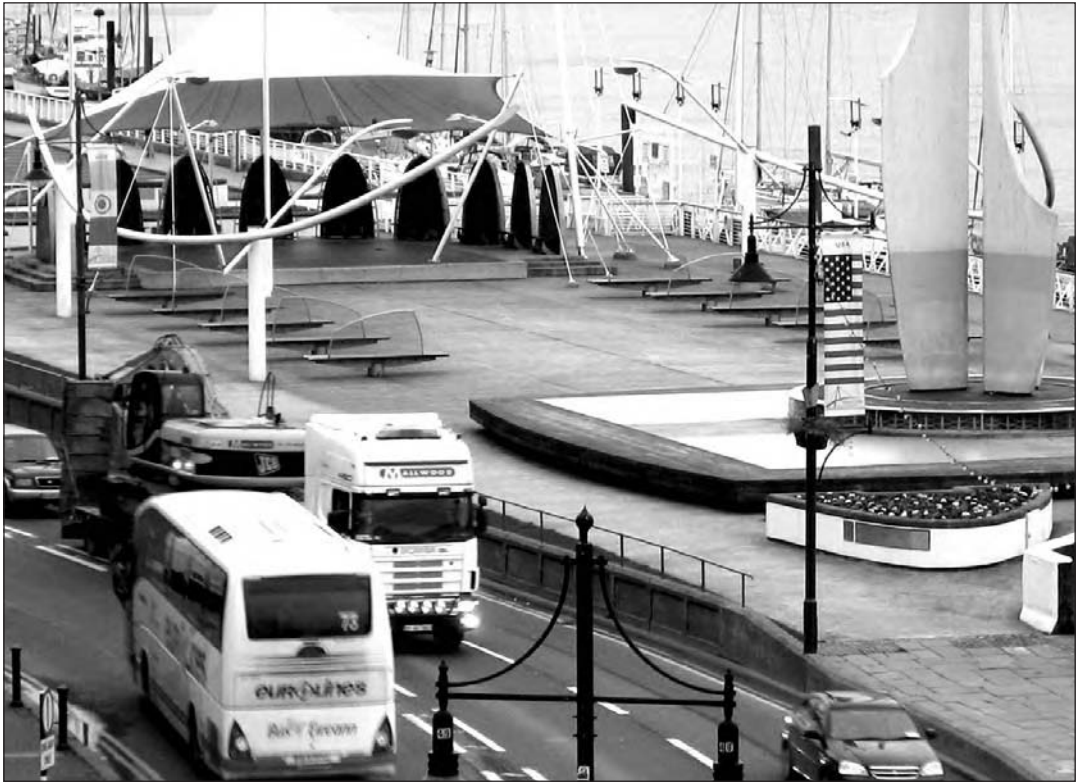
Figure 83 Waterford, Ireland: reclaimed public space by the river, but rather isolated by the adjacent busy traffic artery
