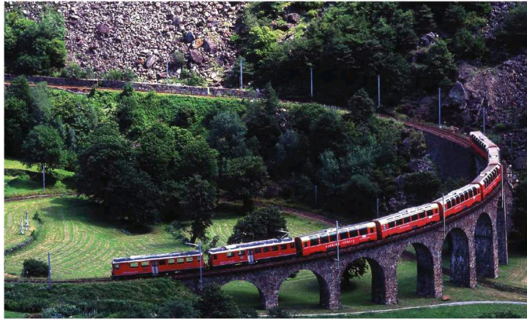
THE BRUSIO SPIRAL VIADUCT IN SWITZERLAND WAS BUILT IN 1908. IT DESCENDS 60FT (20M) AT A GRADE OF 7 PERCENT.
