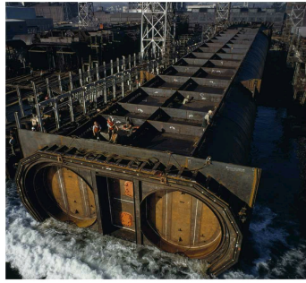
BART TUNNEL SECTION UNDER CONSTRUCTION
