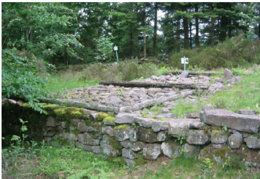
A section of the surviving circuit of the Camp Celtique de la Bure, Saint-Dié-des-Vosges ( département of Vosges). The Gauls were prodigious fortification builders, and the murus gallicus was a peculiar Gaulish type of rampart. It had a wooden framework of intersecting heavy timber beams whose rows were separated by layers of compact earth or rubble. Mortising or long iron nails fixed the beams at each intersection. It was given a cladding of large
