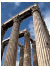
Remaining columns of the Temple of Olympian Zeus
