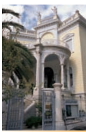
Entrance to the New Wing
