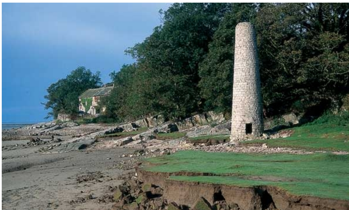
The shoreline chimney at Jenny Brown's Point, Silverdale
