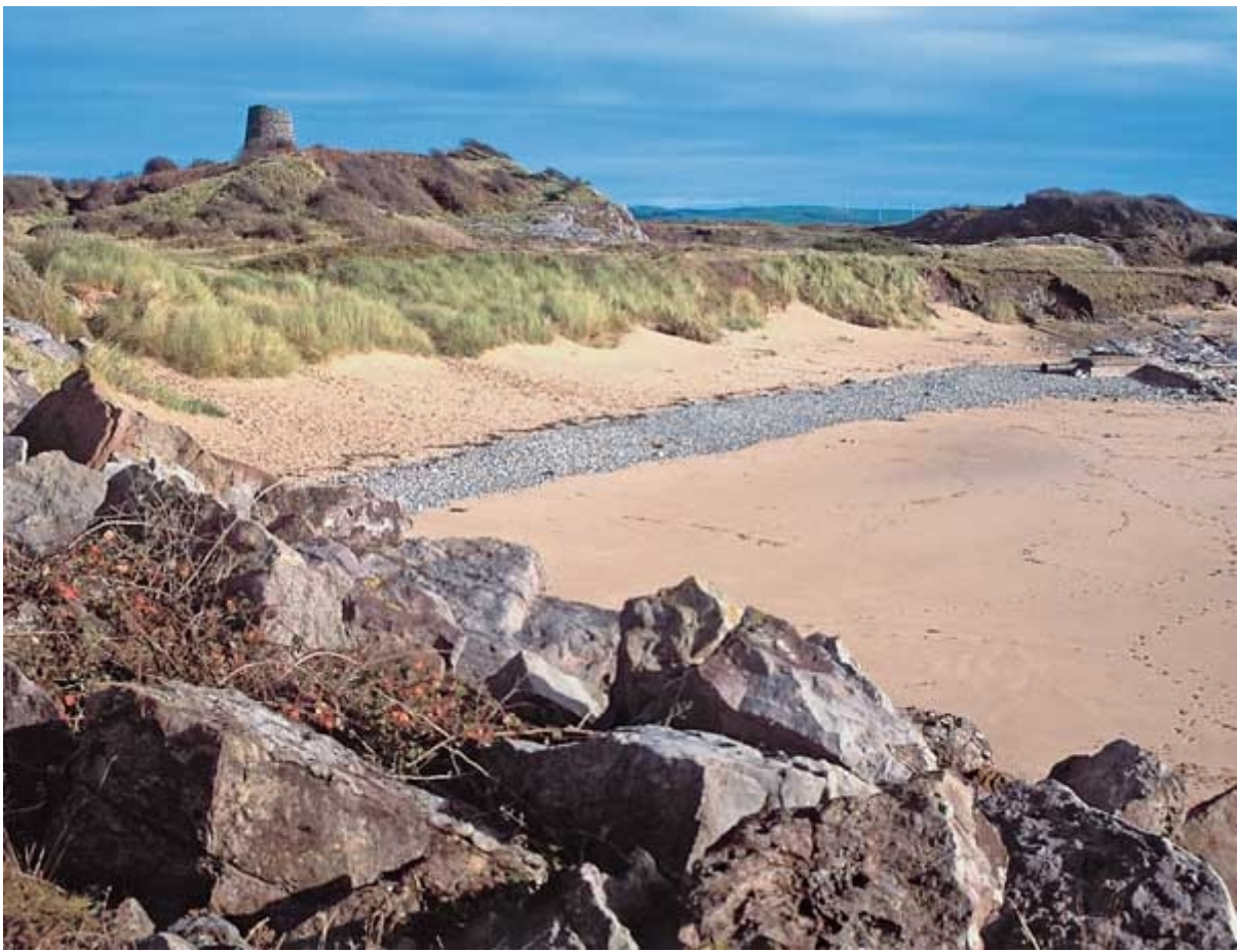
The original lighthouse and the start of the barrier at Hodbarrow Point
