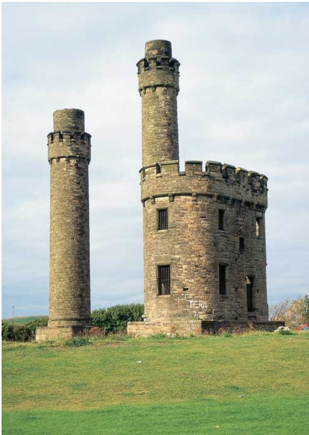
The remains of the buildings of Jane Pit, Workington
