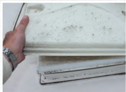
To only wash the unit, remove the four screws and washers, then take off the outer cover
