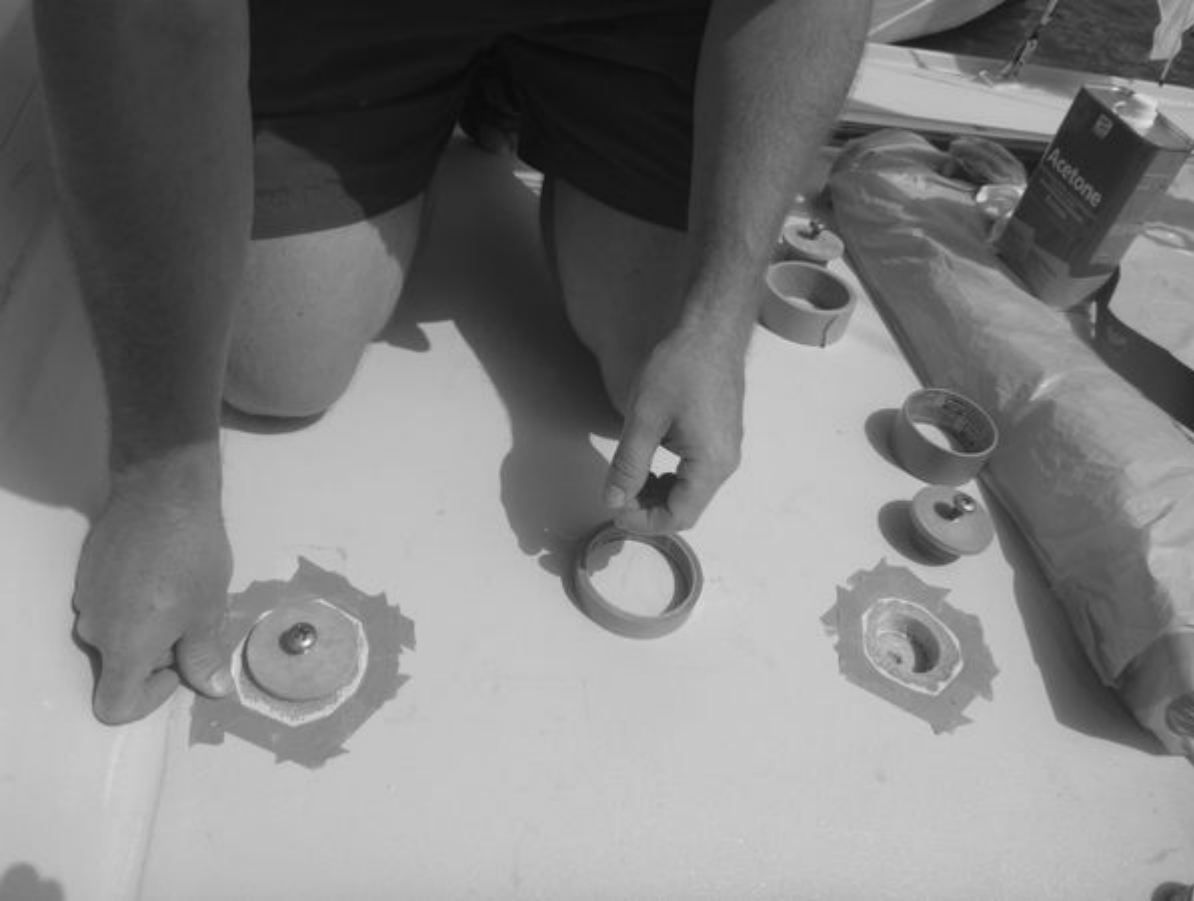
Masking off the wells
