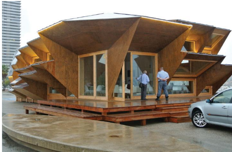
Northwest and southwest facades.
