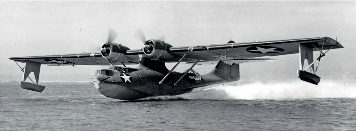
An unidentified PBV gets 'up on the step' during its take-off run. The PBV's wing was mounted high up on a streamlined pylon, keeping the twin engines on the leading edge well away from the water. The outboard floats folded up to form the wingtips.
