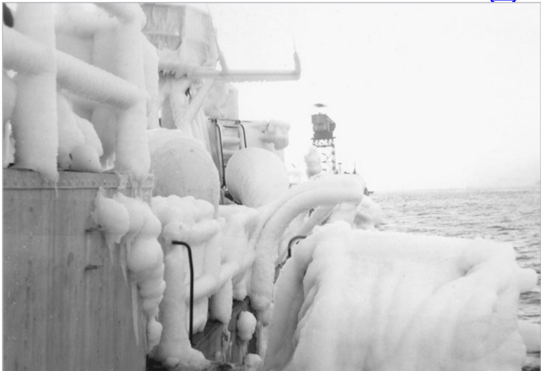
Trentonian entering Halifax harbour on March 3, 1944. This picture is looking aft from the break of the fo'c'sle; the ship is completely covered in ice.
