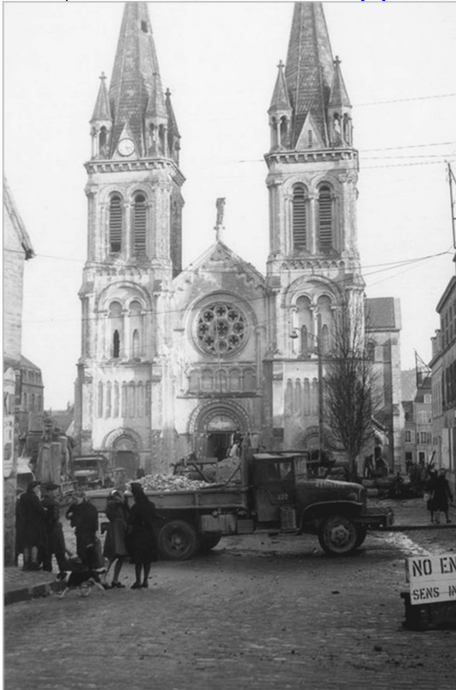
Entry to the cathedral in Cherbourg was restricted while the debris from the recent battle and liberation of the French port was removed.
