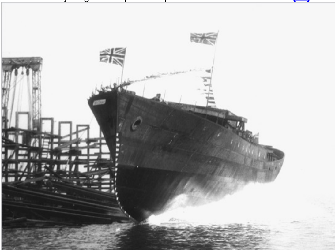
Trentonian sends a large wave across Kingston harbour as the ship enters the water for the first time.
