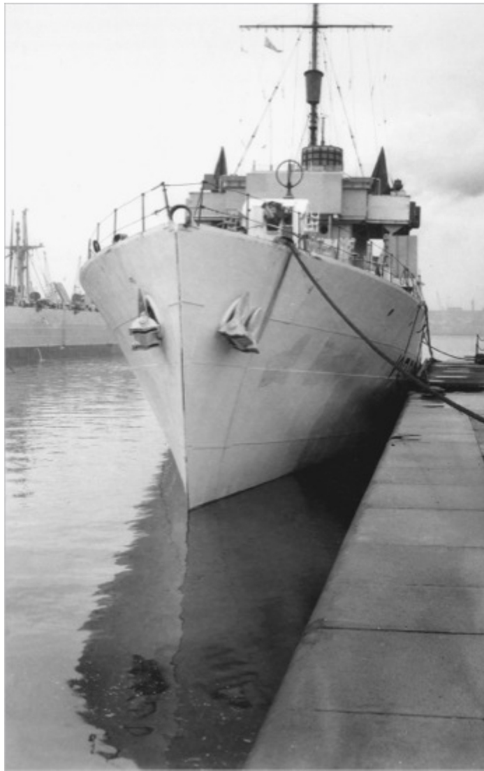
HMCS Trentonian in Cardiff for boiler cleaning, October 1944.
