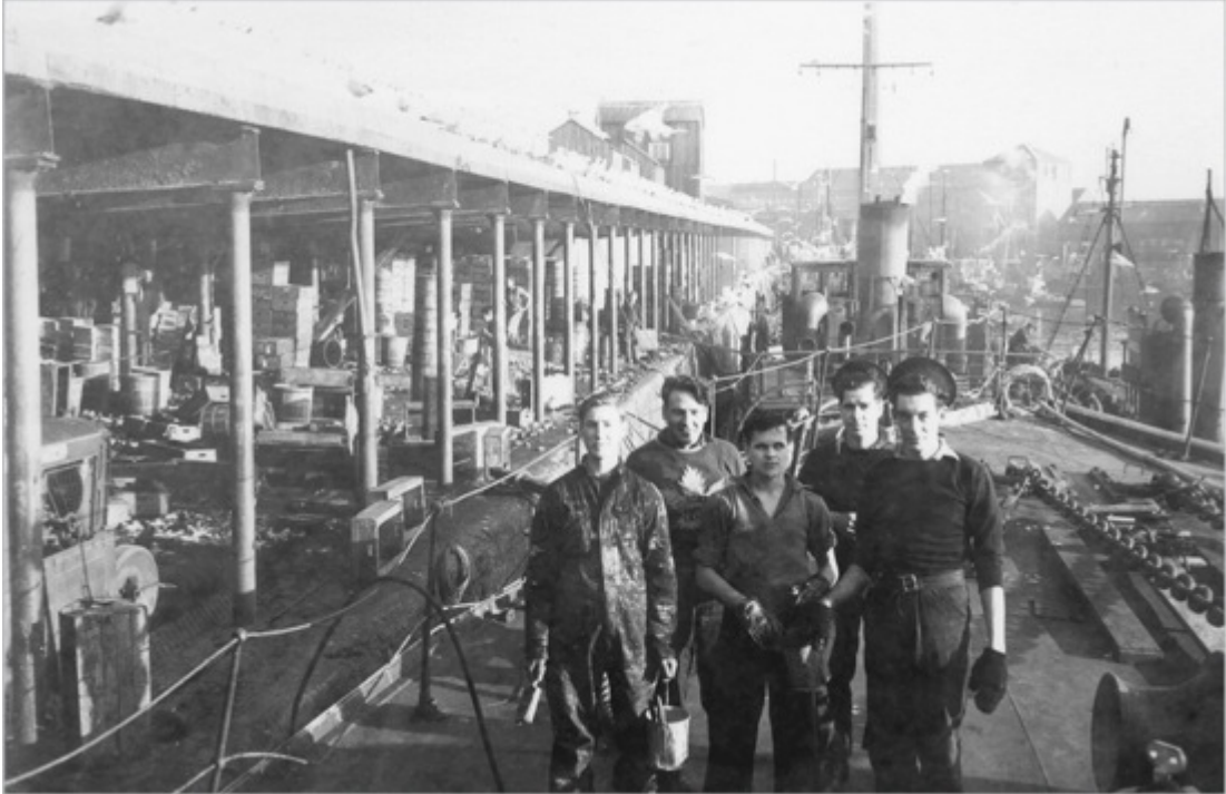
A work party, with a Maple Leaf fan, from Trentonian takes a break during boiler cleaning in Milford Haven.
