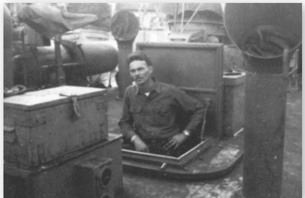
The engine room hatch of an Elco boat amid ventilators and ready ammunition lockers. Over one of the ready lockers is a canvas-covered .50-cal. machine gun on a pedestal mount.
