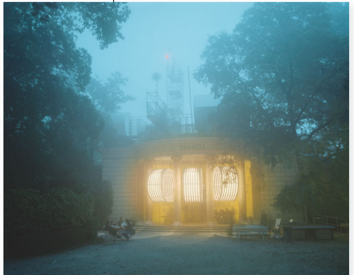
EXYZT, Metavilla, French Pavilion for the Venice Architecture Biennale, Venice, 2006 Shown under construction, the scheme was conceived both as a collective building and living experience within the context of the exhibition and as an embassy for French design.
