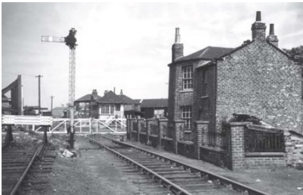
Stockton Toll House, seen around 1970 before the tracks were taken up, was one of three designed by John Carter in classic turnpike fashion. Each had a wagon-weighting machine so that the appropriate toll could be calculated.
