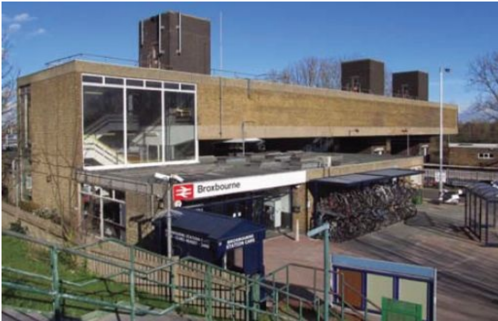
Broxbourne (Peter Reyniers, 1960). Through the entrance-hall window we see the robust concrete bridge deck. A vertical accent, emphasised by contrasting brick, is provided by the lift towers, originally intended for parcels movement.
