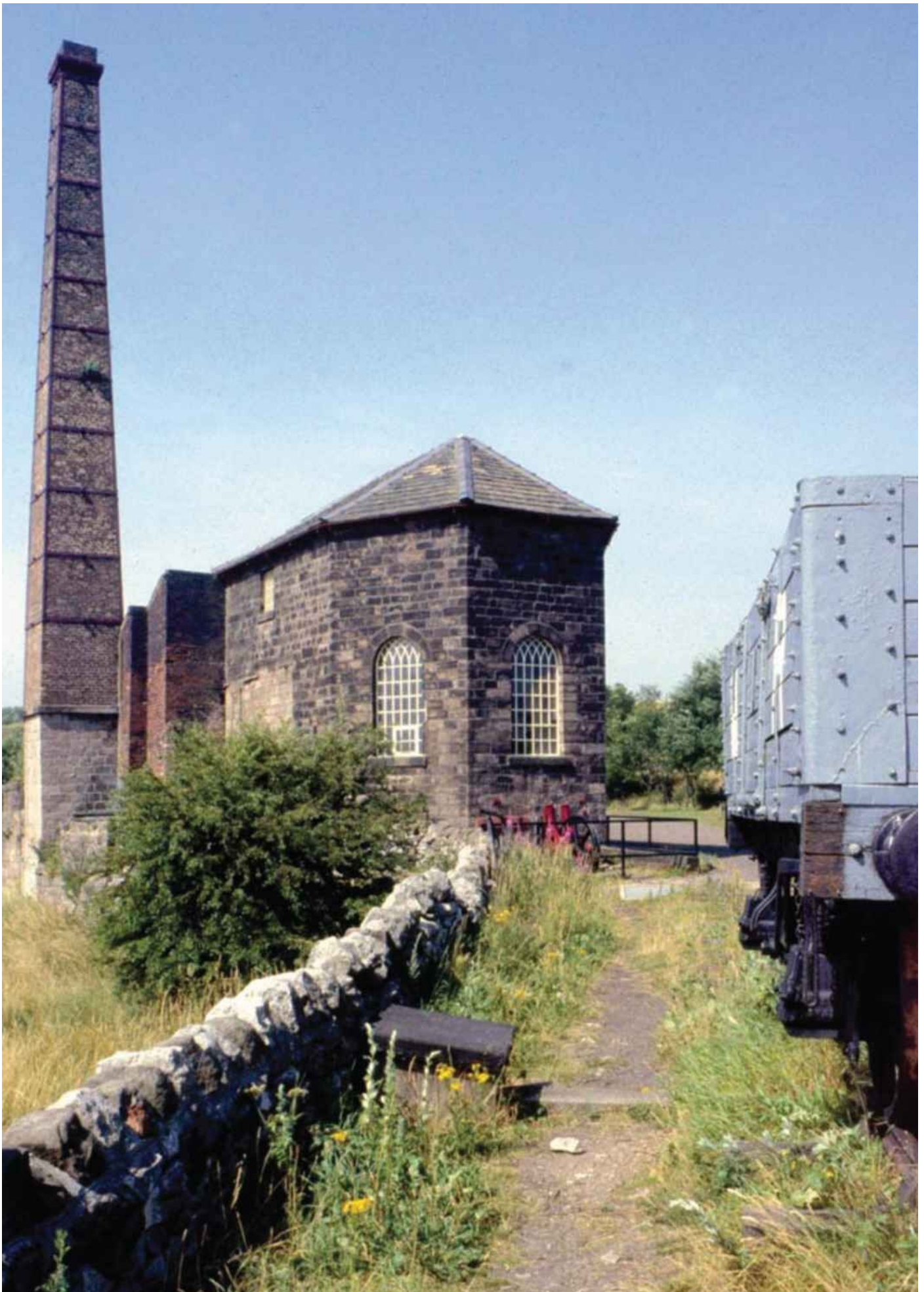
Middleton Top engine house, Derbyshire, was preserved following closure in 1963 and retains the two-cylinder beam engine supplied in 1829, albeit with many parts
