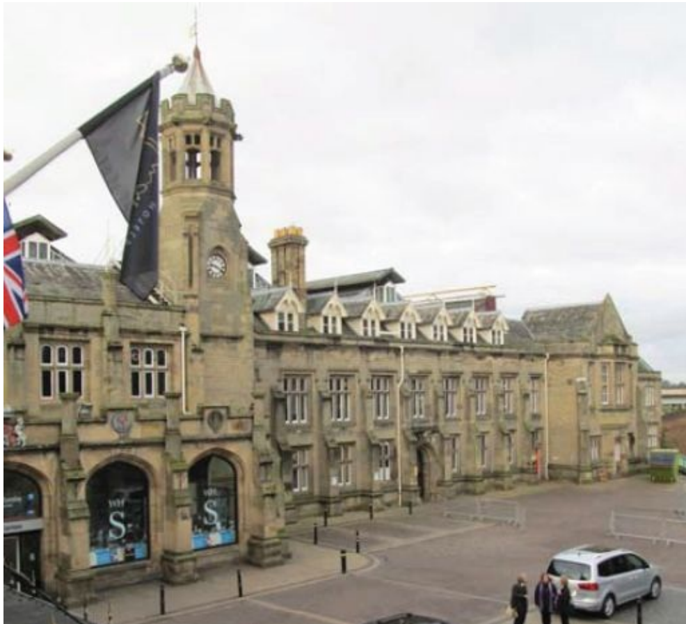
Carlisle: Tite's 1847 office range now fronts an impressively large and light trainshed of 1881, whose gables can be seen poking up behind.
