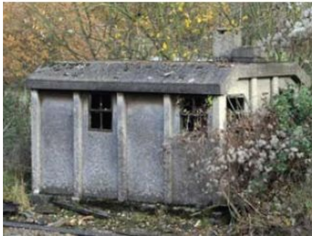
Wayside concrete. A gate-keeper's cabin built with the LNER system of concrete panels slotted into upright posts, and a Southern platelayers' hut.
