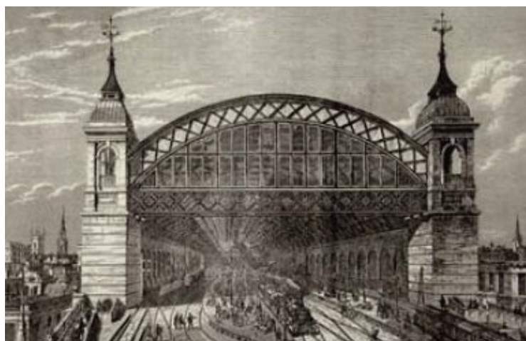
Rarely does a station's rear attract more prominence than its front, but London's Cannon Street (1866) faced over the Thames, so the trainshed was framed by towers, which are the only notable features to survive rebuilding after war damage.
