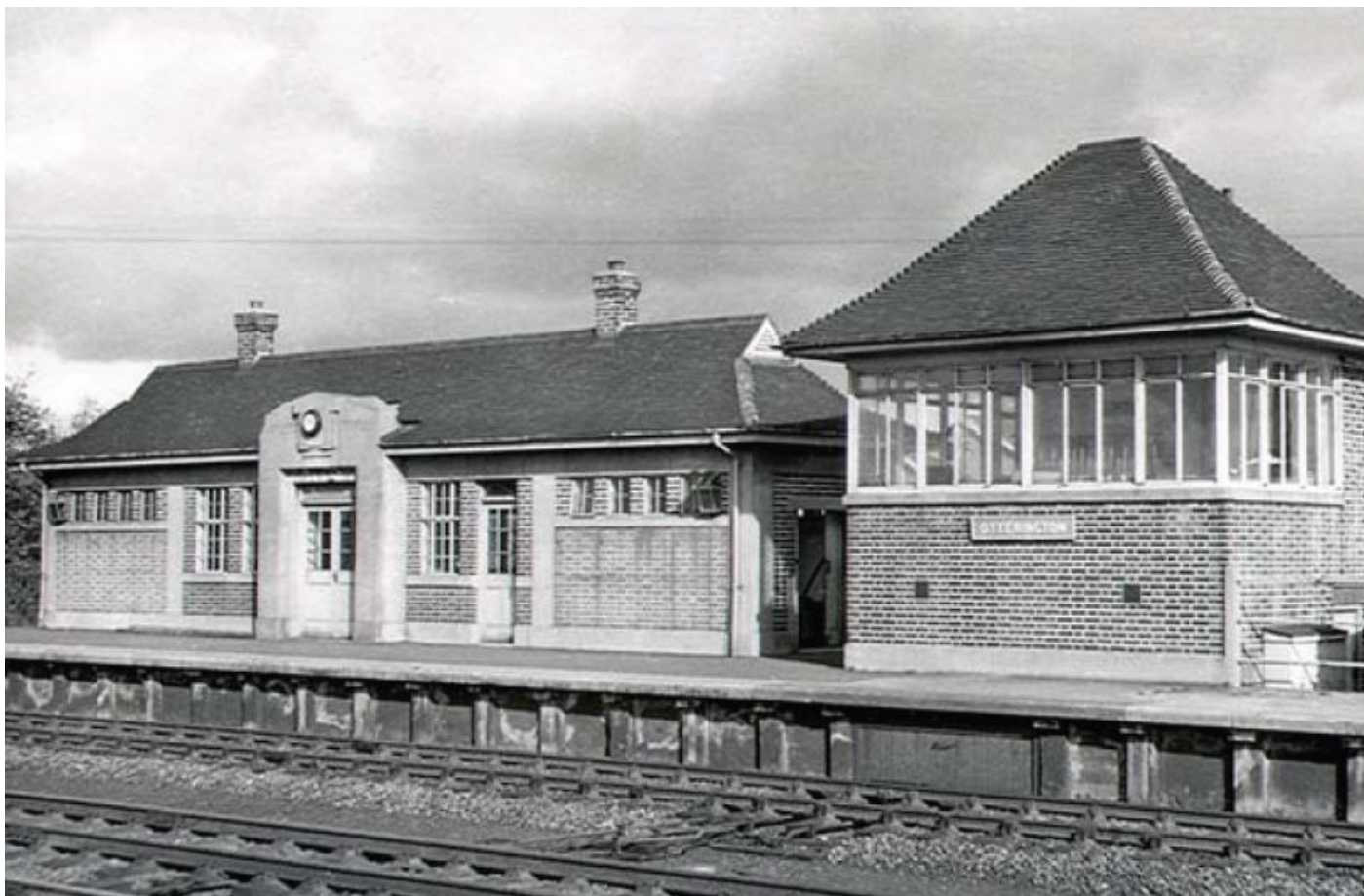
Otterington station and signalbox: a carefully detailed essay in modernised-Georgian manner by Robert Darling of the LNER York office. The small-windowed ends housed a lock-up store and toilets, the centre an office and waiting room.
