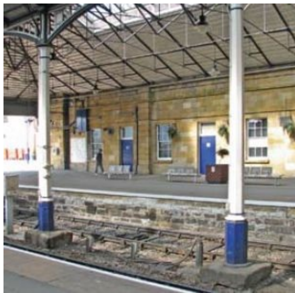
The Euston-style trainshed at Scarborough (George Townsend Andrews, 1845). The columns sit on stone blocks that have been exposed by lowering the tracks to obtain higher platforms.
