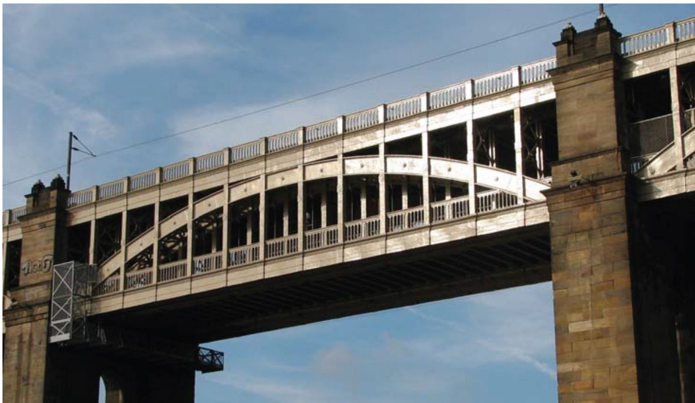
Newcastle's High Level Bridge has an architectural quality deriving from its enclosed form, with the railway borne on cast-iron arches, and a roadway hanging from them.
