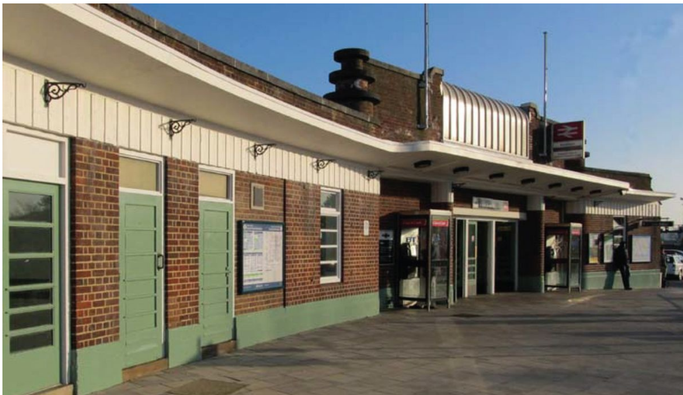
Horsham. The parcels office and footbridge have a feature entrance off to the left, from which a broad corridor curves round the station front to the booking hall and main entrance.
