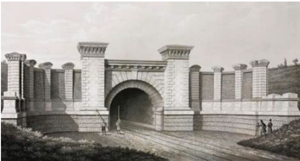
Primrose Hill Tunnel, London: east portal (1837). The artist has introduced a surveyor, right, taking a sighting on to the tall pole, to emphasise the engineering involved. A second tunnel, with matching entrance, was built alongside in 1879.
