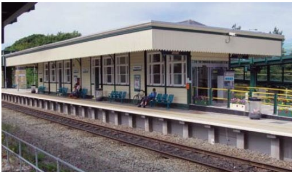
Prestatyn is a well-restored example of LNWR modular wooden buildings with their distinctive tripartite windows. The platform has been rebuilt with the precast concrete components commonly used since the 1930s.
