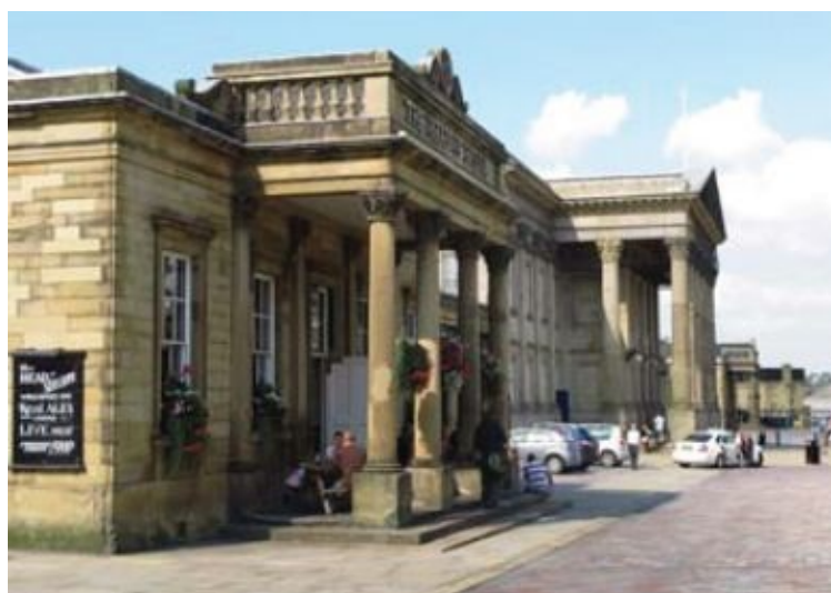
Huddersfield: the nearer portico was the entrance to a booking office, marked by company heraldry above the parapet. The trainshed, of no particular distinction, was replaced by the present, larger one in 1886.
