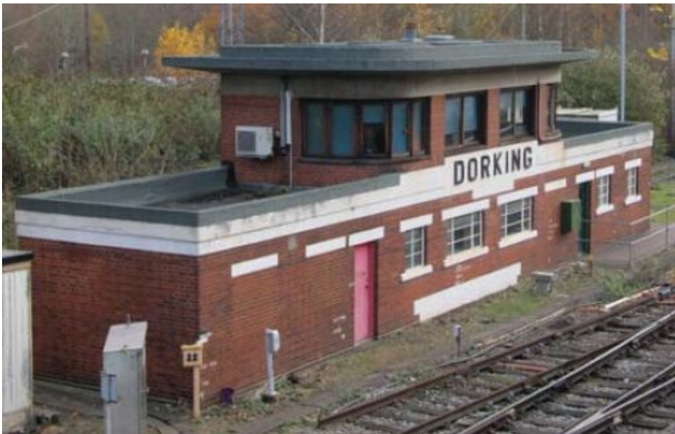
Dorking (Surrey) signalbox dates from 1938 and is a good example of the Southern's Moderne style. Where these boxes were sited between running lines the operating floor was bow-ended, with windows wrapping right round, as at Wimbledon.
