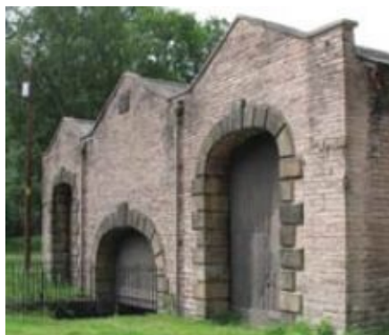
Whaley Bridge, Derbyshire. Integrated transport: the warehouse provided shelter for transhipment between a branch of the Peak Forest Canal and flanking railway tracks that entered through the two big arches.
