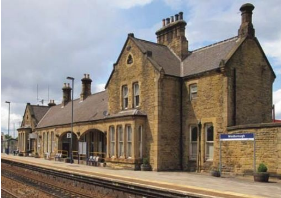
Mexborough. A stone arcade on cast-iron columns featured also at the North Eastern's Rowley station (William Peachey, 1873, with handsome barley-twist columns), which has been re-erected at Beamish Museum (County Durham).
