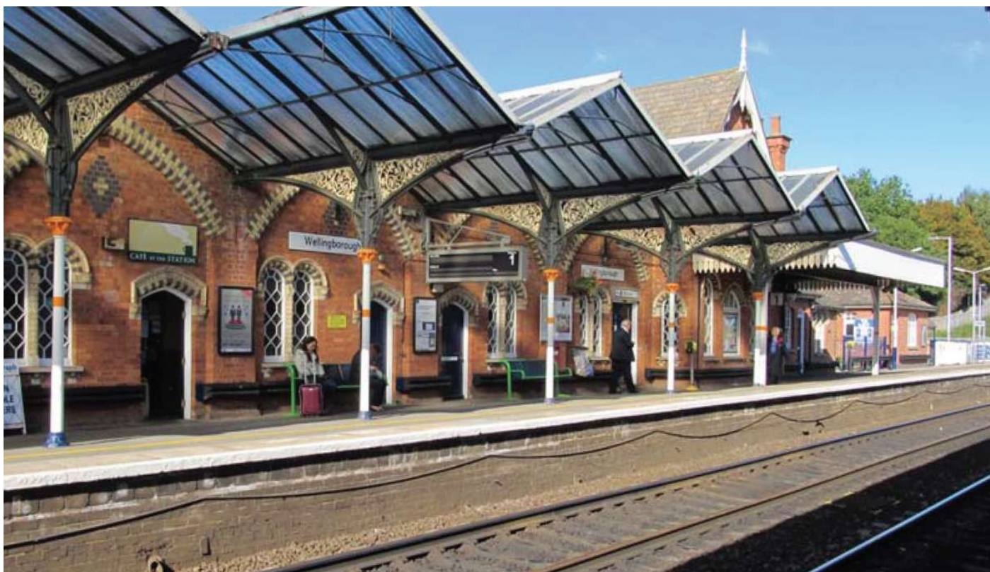
Wellingborough's verandah originally had filigree ironwork in the open gable ends. A comparable roof survives at Kettering, though its accompanying building has been replaced.
