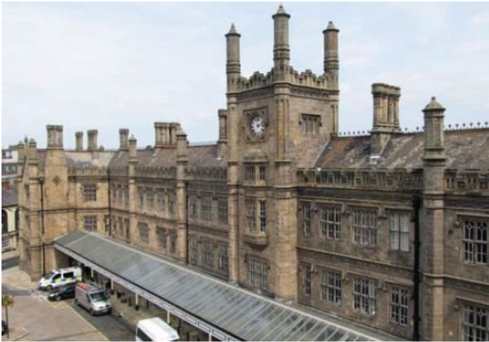
Shrewsbury's canopy eaves mark the original ground level, which sloped down to the far end, where Penson added the three-storey wing in 1855. The rest of the building was dug beneath and underpinned for today's ground floor in 1903.
