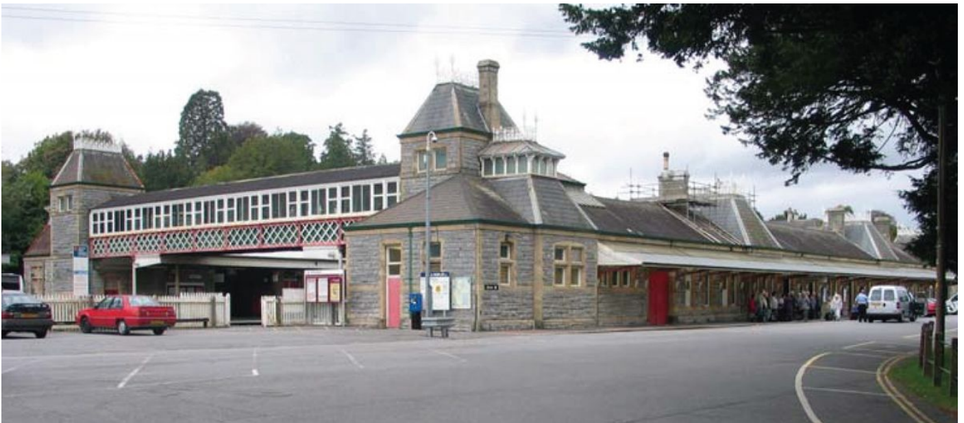
Torquay station was rebuilt in local limestone, with the iron-crested pavilion roof stepping gracefully up into the footbridge tower. Tiverton, built shortly afterwards (1885), was similar but with gabled roofs; it has been demolished.
