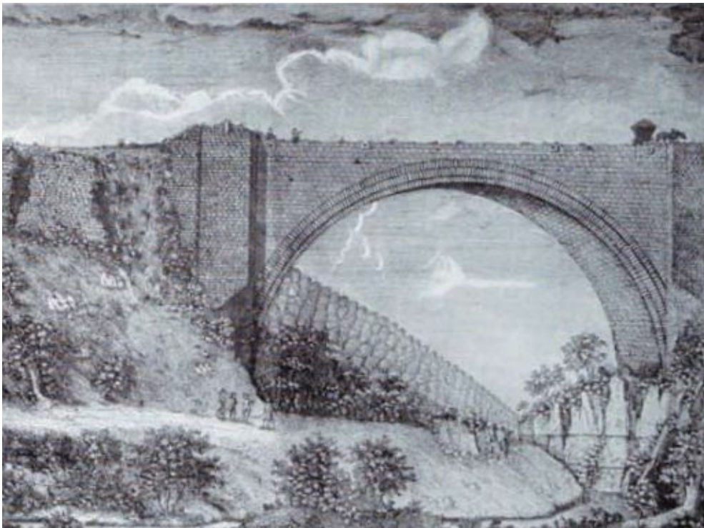
Causey Arch near Stanley, County Durham, was built in 1727 for the Tanfield wagonway. Its 32-metre span, then the largest stone arch in Britain, emphasises the profitability of some early wagonways.
