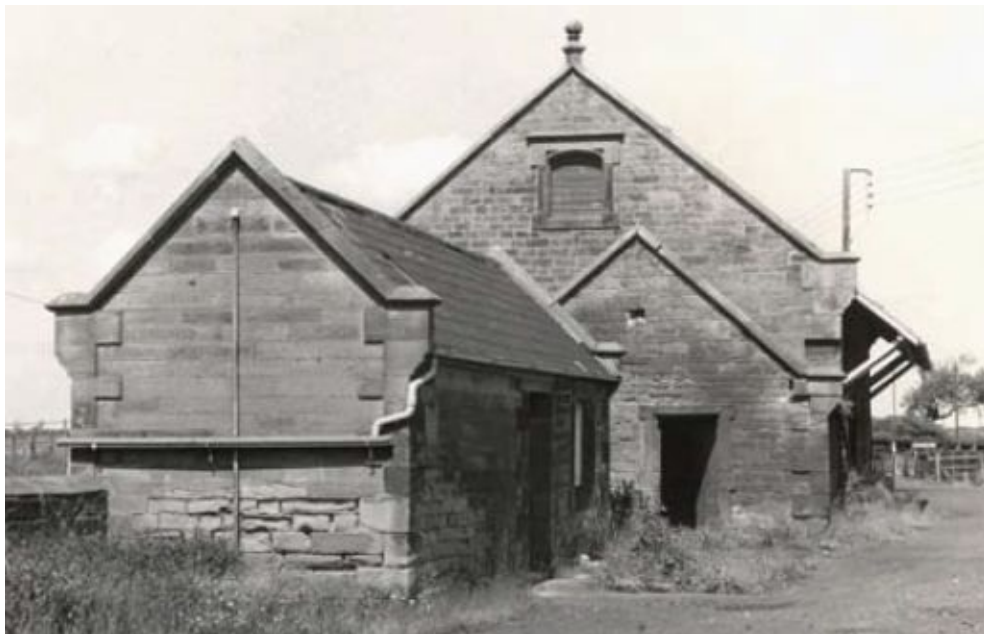
Acklington goods shed, Northumberland (1847, recorded 1973, now a dwelling). Benjamin Green designed this to match his Jacobethan station, a style maintained in the later stable, whose open door beckons.
