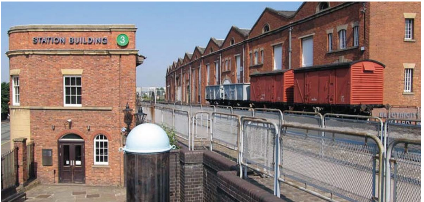
Manchester Liverpool Road terminus, now the Museum of Science and Industry; on the left is the passenger station, with the carriage shed at this end; the goods warehouse is on the right.
