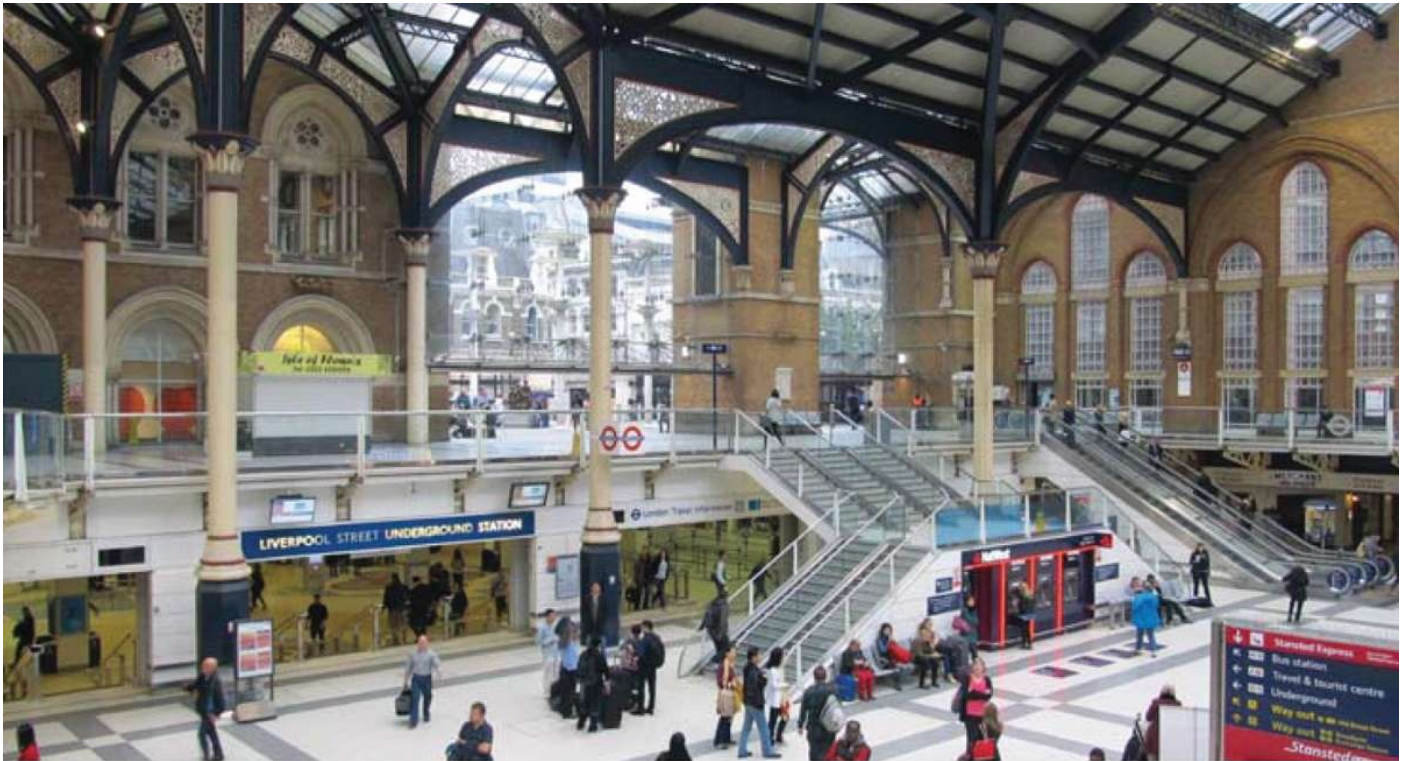
Liverpool Street: the 1991 concourse and roof. The platforms are below street level, where a mezzanine gallery serves a line of shops, in modern glass tunnel idiom, which define the concourse edge without compromising the vistas through the trainshed.
