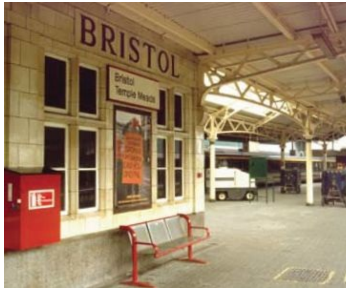
Bristol: the new platforms of 1935 feature almost identical buildings to Cardiff, faced in Carrara-ware faience with moulded lettering in GWR chocolate.
