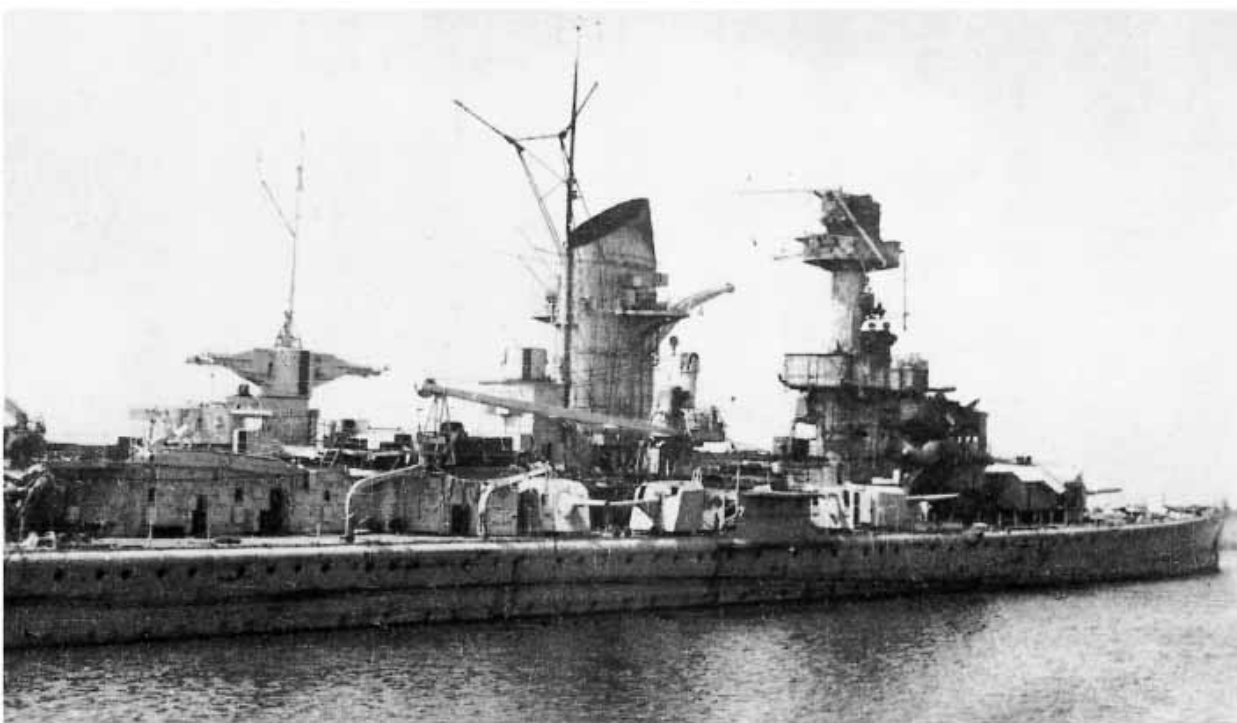
The wreck of Liitzow photographed at Swinemünde shortly after the capitulation. Having expended her remaining ammunition to bombard Soviet forces from mid-April, the cruiser was abandoned, but she survived a scuttling attempt by explosives on 3/4 May 1945. Her subsequent whereabouts are unknown.
