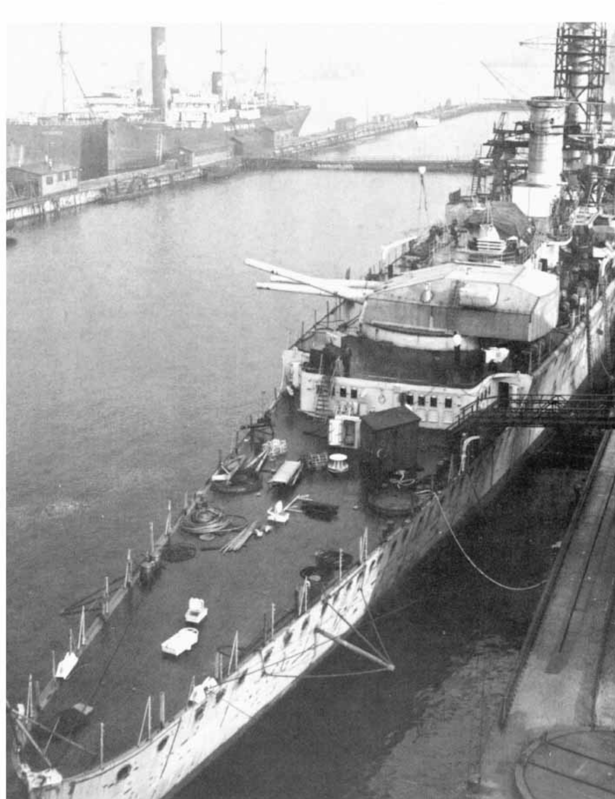
A stern view of Deutschland nearing completion. The quarterdeck lacks only the two banks of torpedo tubes, the rotating bases for which are visible. 'B' turret is trained to starboard, probably for testing purposes. Staging is still present around the battle-mast and funnel. Notice the armoured window blinds on the rear bulkhead of the forecastle deck. Both propeller guards have been extended.
