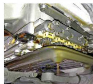
Here's the valve body with the gearbox sump removed.
