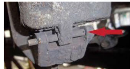
The clip was missing from the brake pad retaining pin.
